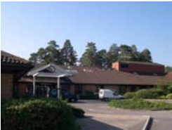
Chase Community Hospital - Bordon
