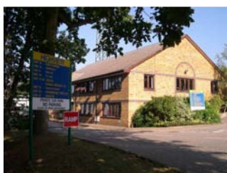
More quality units like these, built in 1990, at Highview Business Park are desperately needed to expand business in the town
